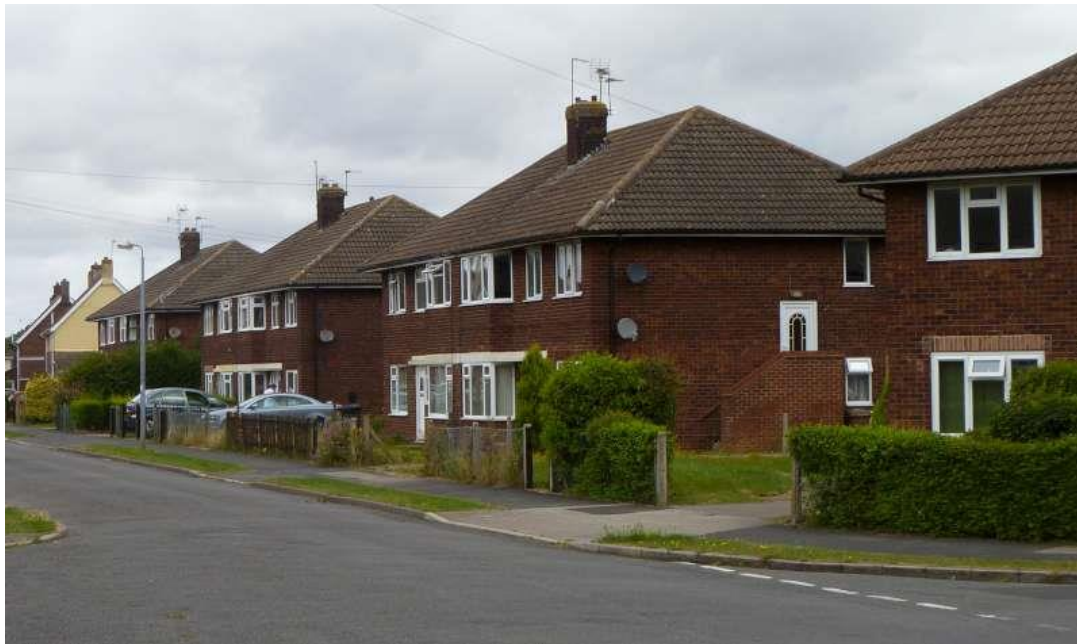
80. Grange Road flats
