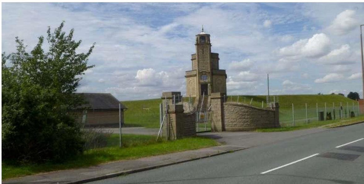
34. Pump House (Water Tower) Grantham Road
