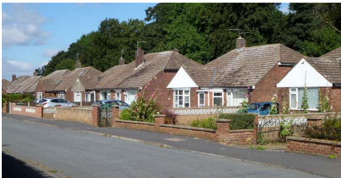
42. Churchill Avenue showing hipped roofs
