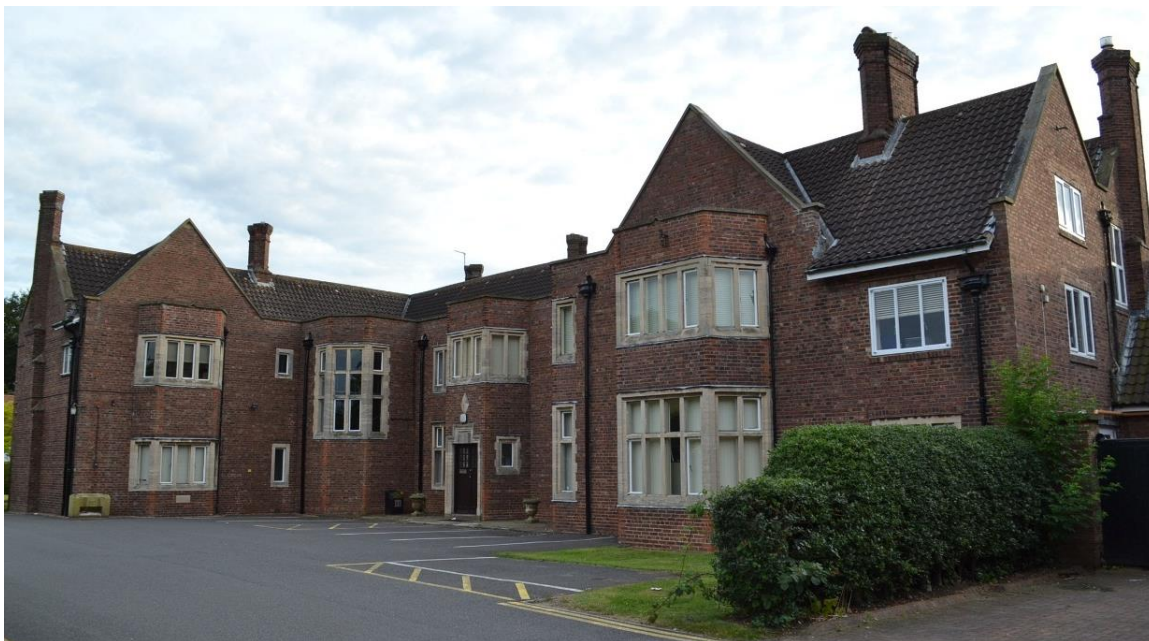
10. Cross o' Cliff Court (Red Hall House)
