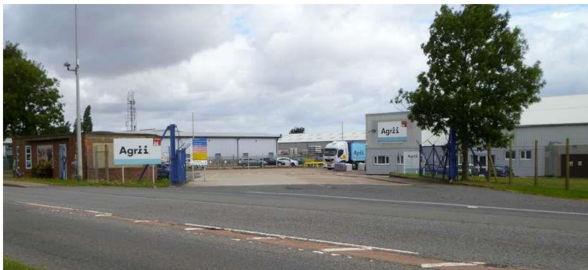
94. Entrance to Agrii showing the wide WWII aircraft entrance and Guard Room on left
