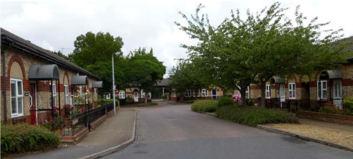
74. Meadow Way terraced bungalows with their brick paved paths and road
